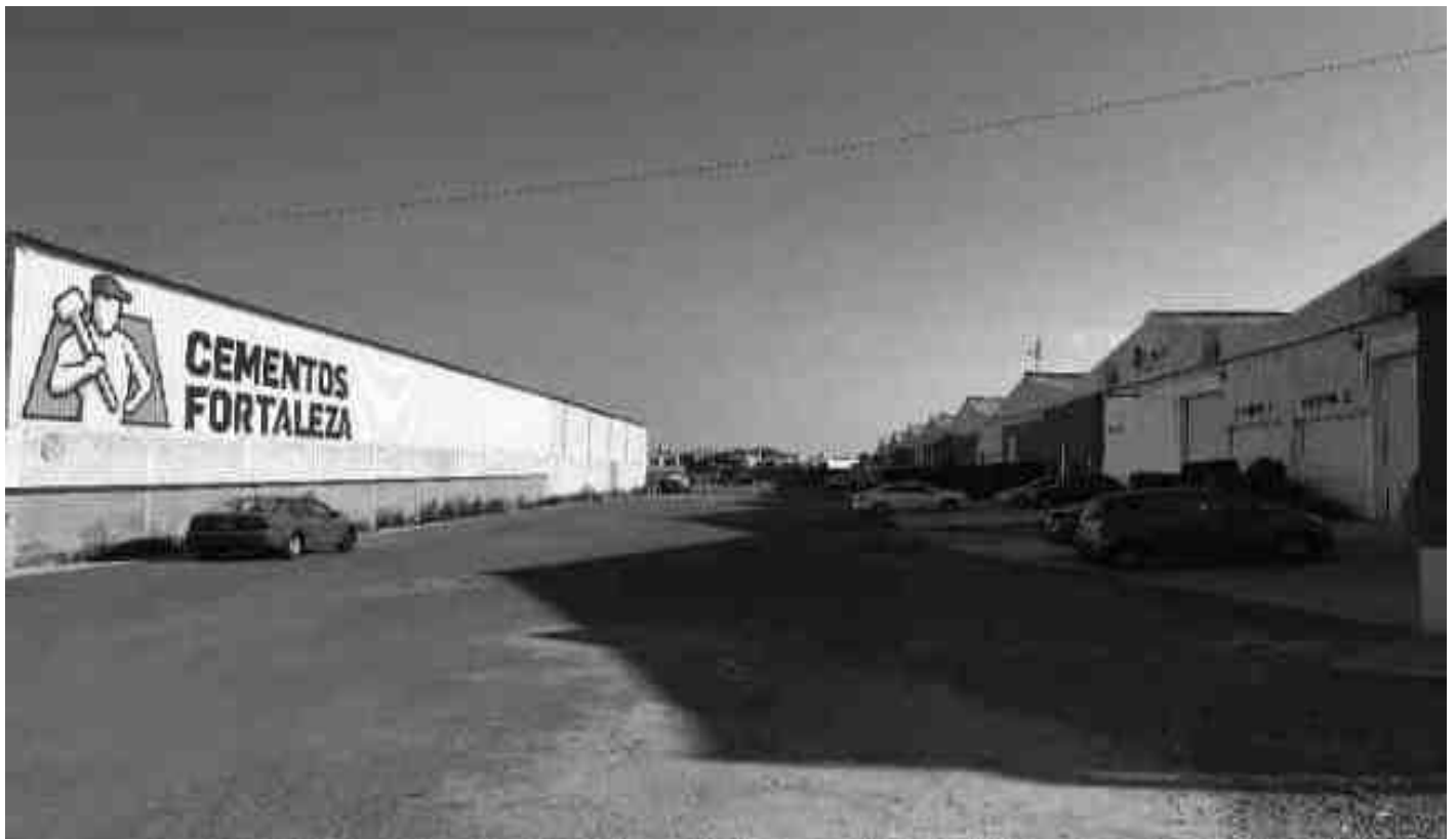
Parte Interior FOAMOTIVE MEX, S.A. de C.V.
